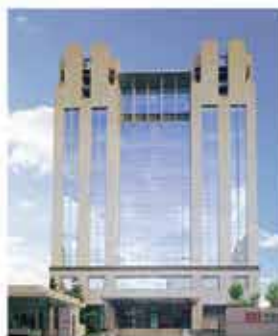
MEAN WELL GUANGZHOU TIANHE R&D CENTER
